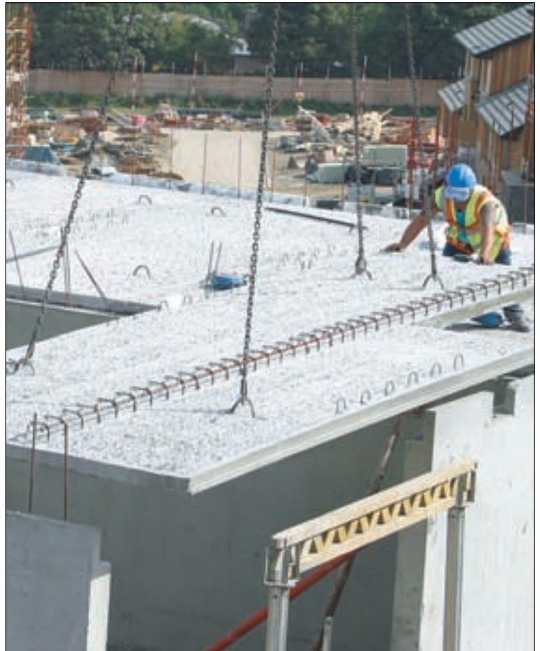
Safe Load Table for Propped Flood Wide Slab, Note: Tabular Values are Spans (m)
